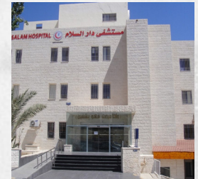
Dar Al Salam Hospital Project - EGYPT
