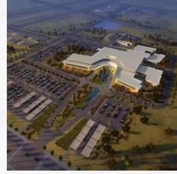
Ministry of Health Project - QATAR
